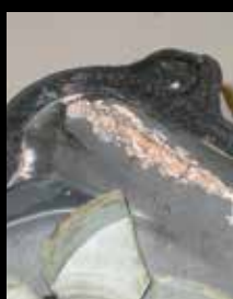
Deposits /Calcium Buildup
